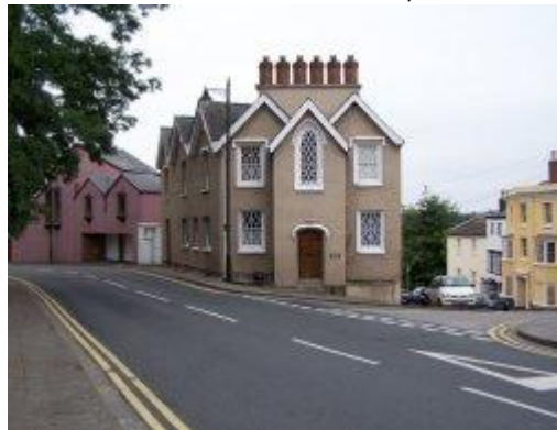
Old Castle Vaults building
